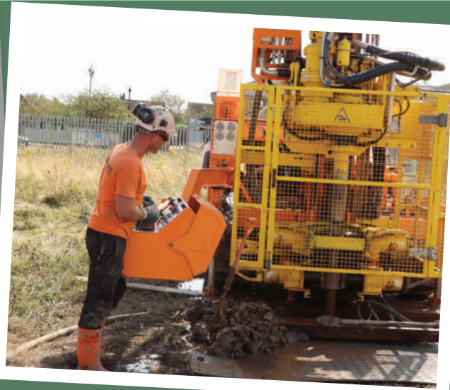
Pictured: Work has begun to make 50-metre deep boreholes into the ground.
