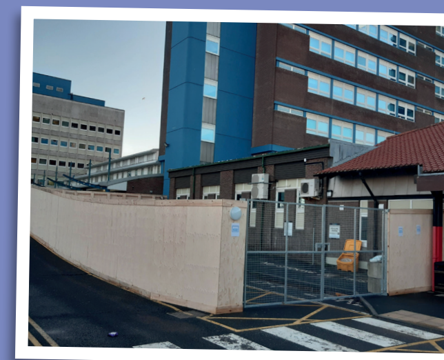
Pictured: The construction access point
