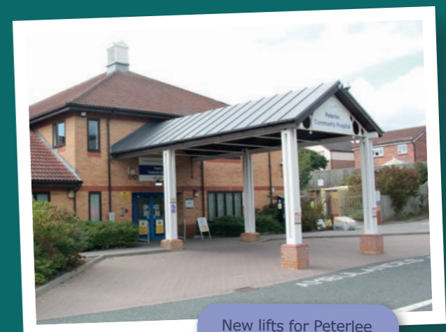
New lifts for Peterlee Community Hospital
